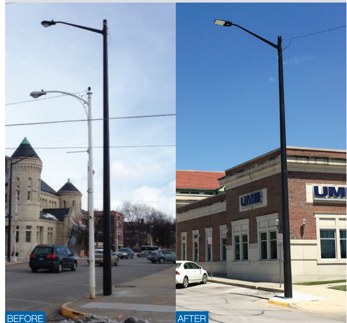
BEFORE Pole on left: Old, rusted steel pole Pole on right: New, durable prestressed spun concrete pole (photo: The StressCrete Group)
